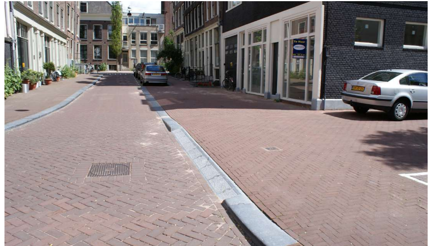
Image 4.4: Example of crossover junction design
