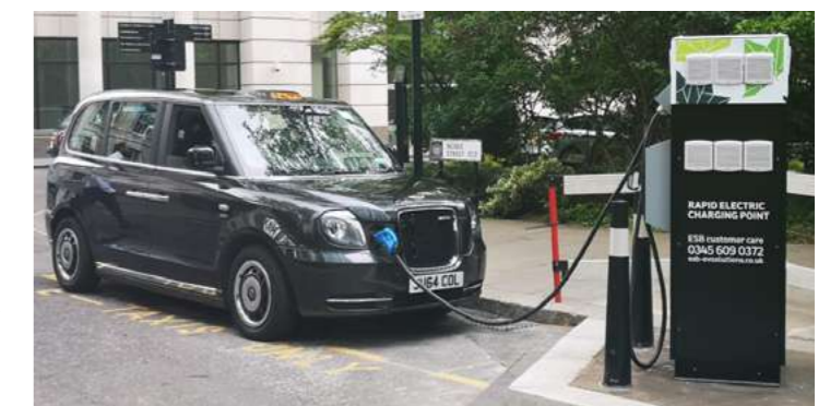
Image 4.7: Example of EV charging point
