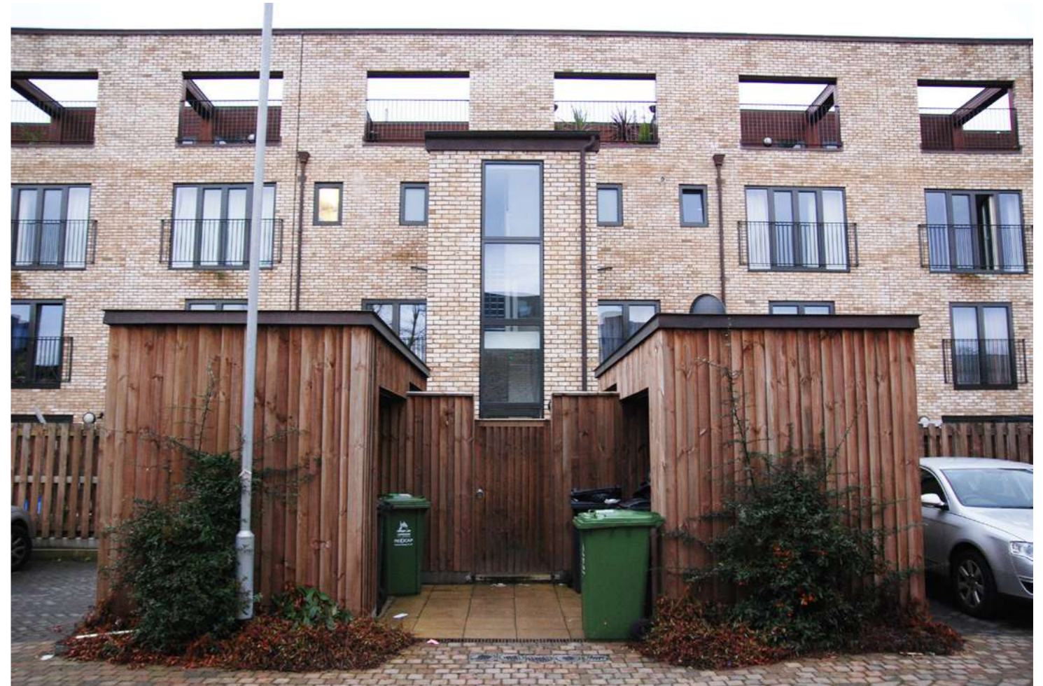
Image 6.6: Servicing is well-integrated into the design of the development within the rear parking court
