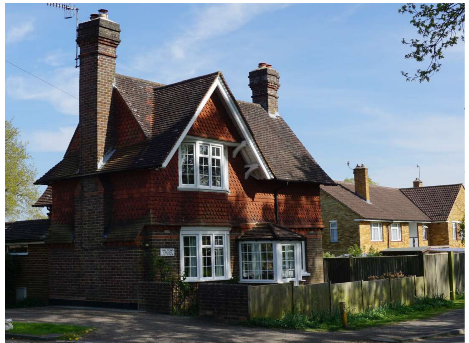
Image 7.3: Stock brick and clay tile hanging
