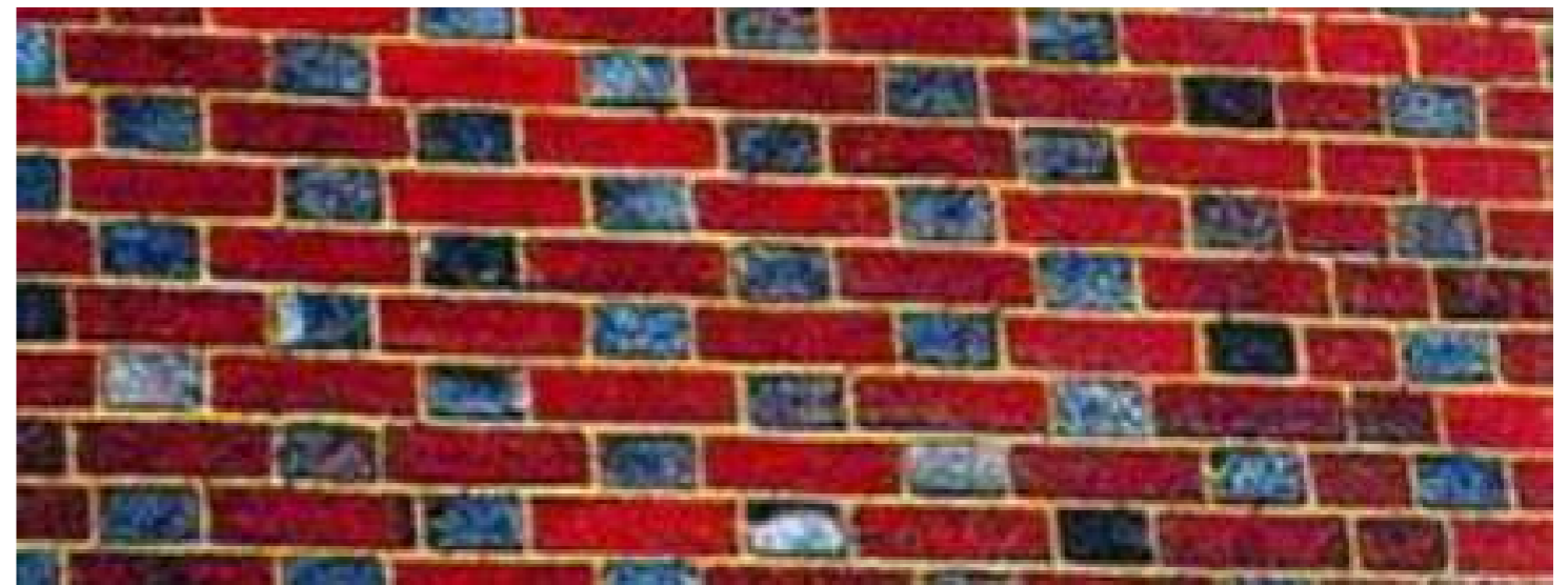
Image 7.2: Flemish bond handmade red brickwork with burnt headers (image from RBBC Character and Distinctiveness SPD)
